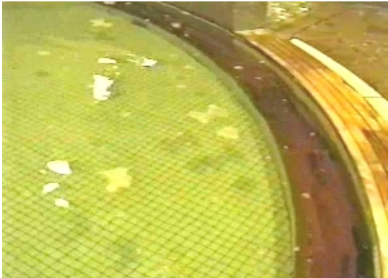
Biofilm removal started within hours after MIOX system start-up
