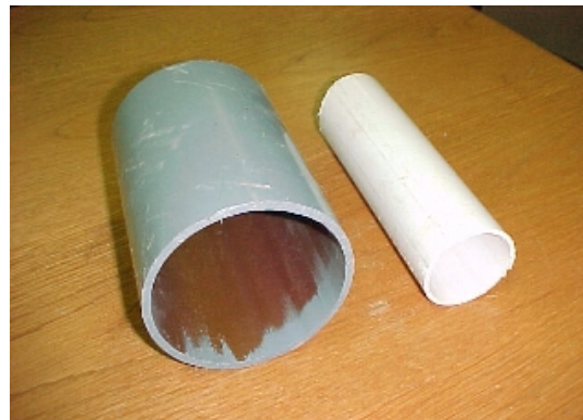
Biofilm contamination on chlorine-treated line (left) versus mixed-oxidant line (right) at Diana Water Supply
